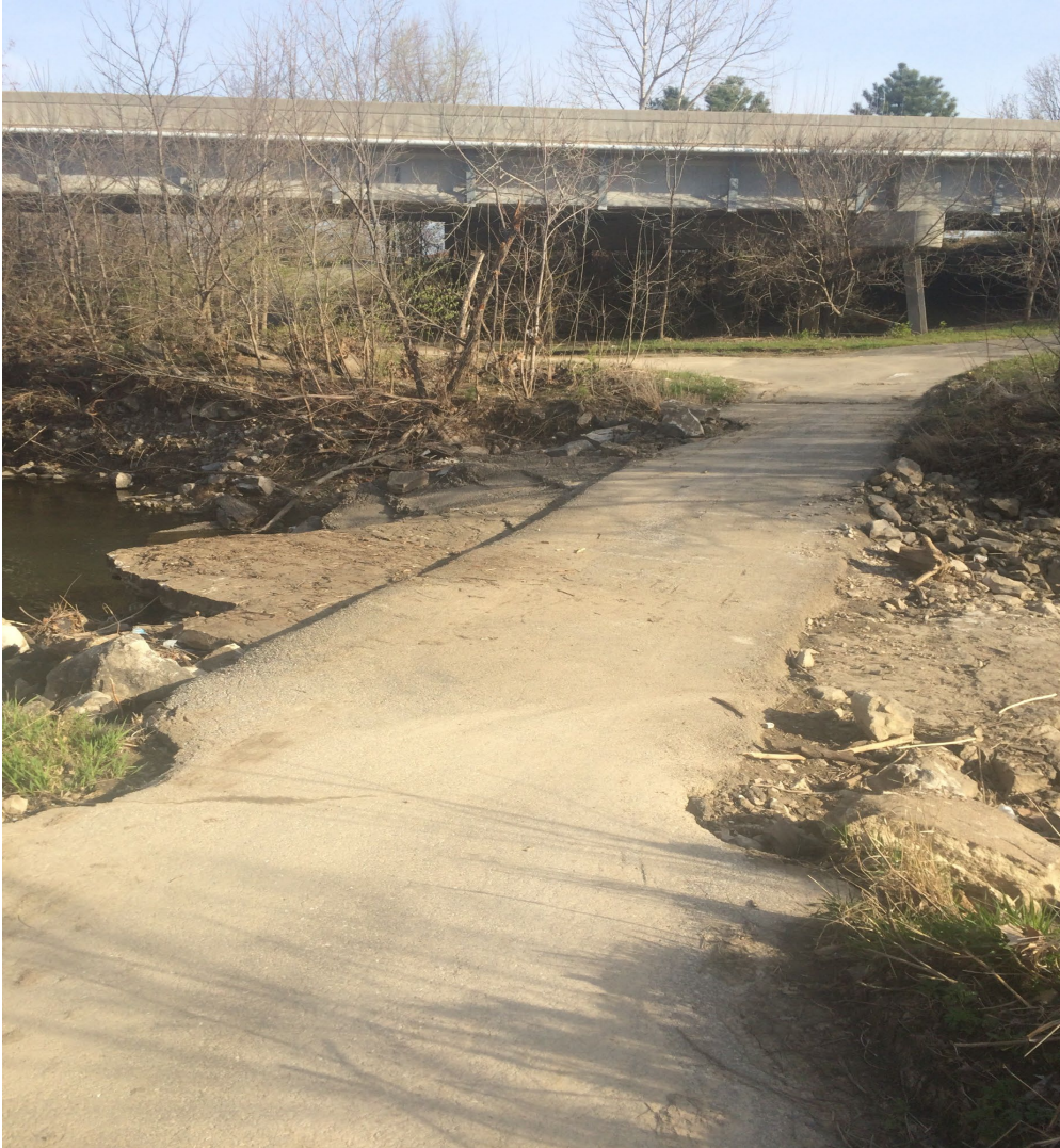
Low water crossing when passable
