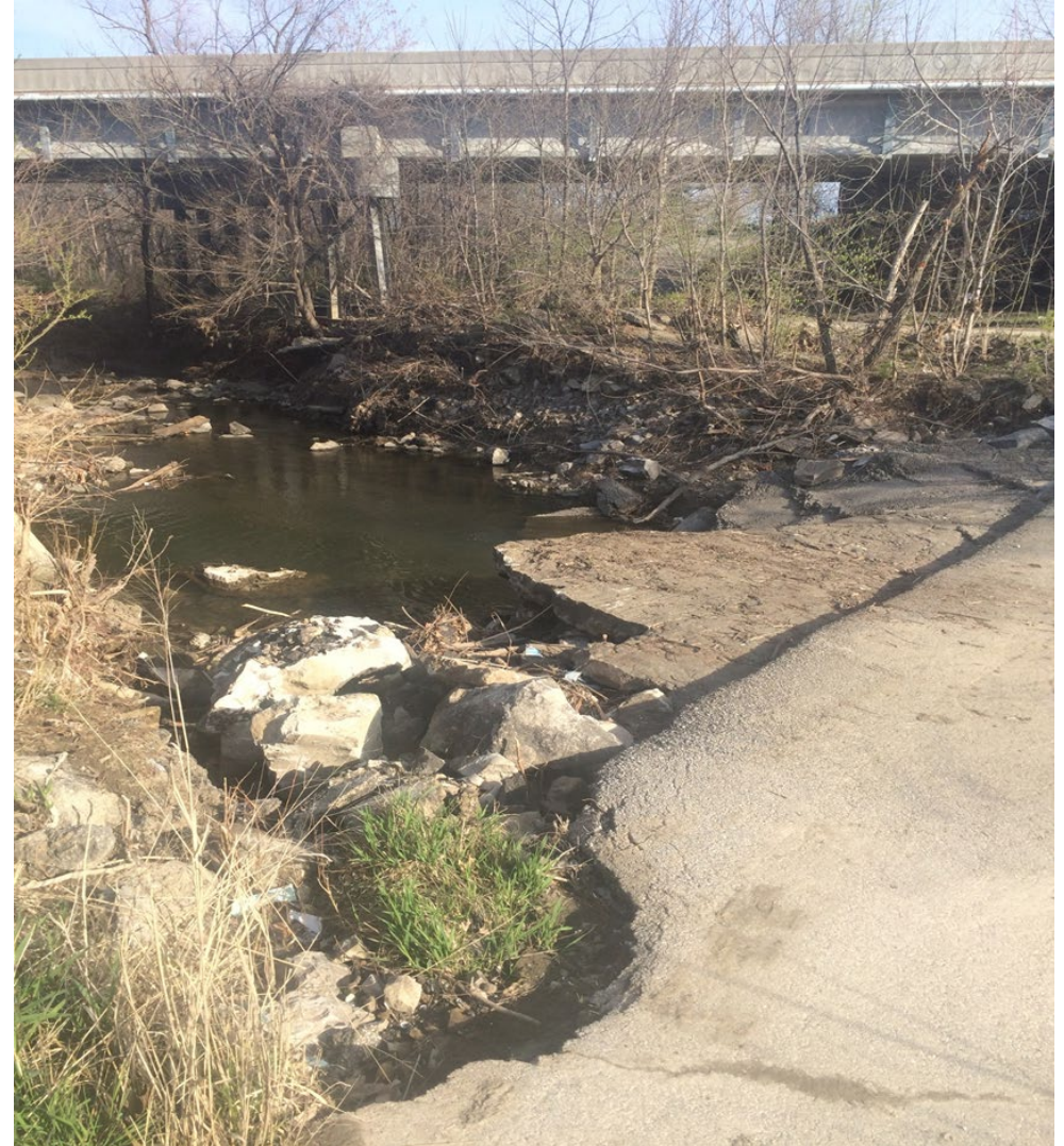
Normal creek flow at low water crossing
